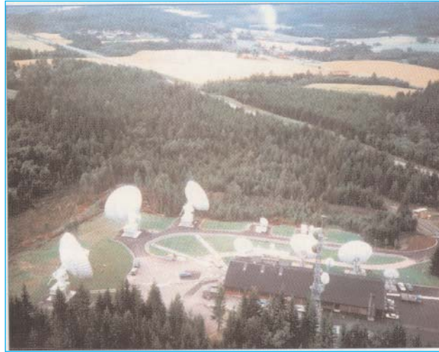
Figure 9 Nittedal earth station outside Oslo, Norway
